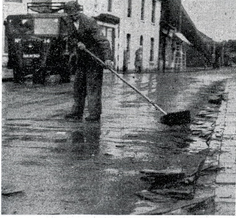
The shop window in Rodbourne Road (top) smashed by a small whirlwind yesterday afternoon. Below, a Corporation employee clearing the debris of smashed roof slates.
