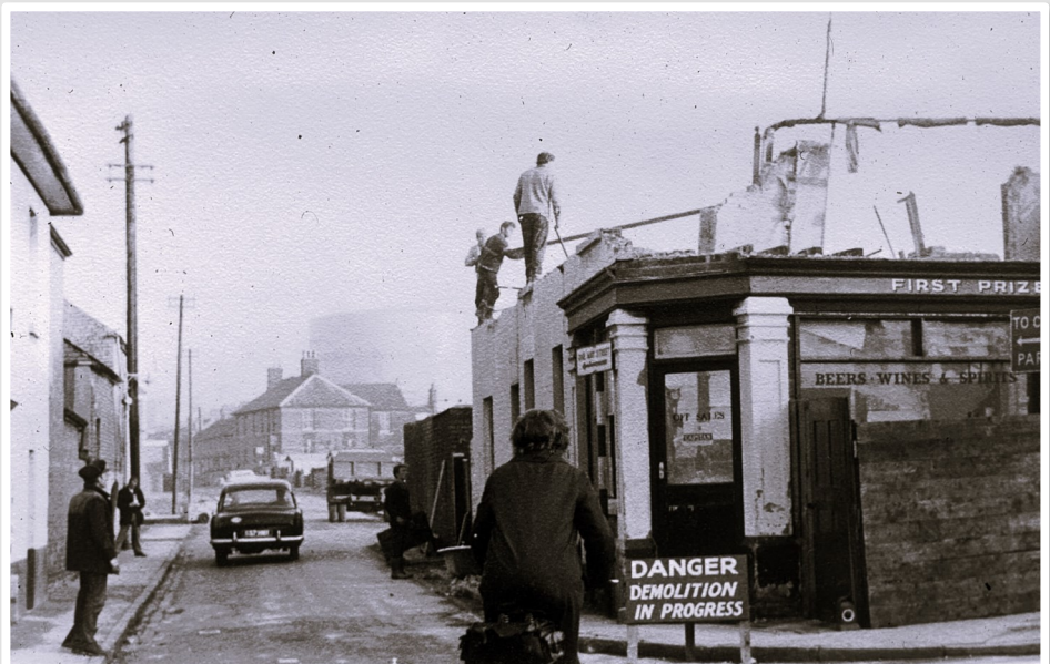
Demolition of the Carpenters Arms, Gorse Hill - 1962
